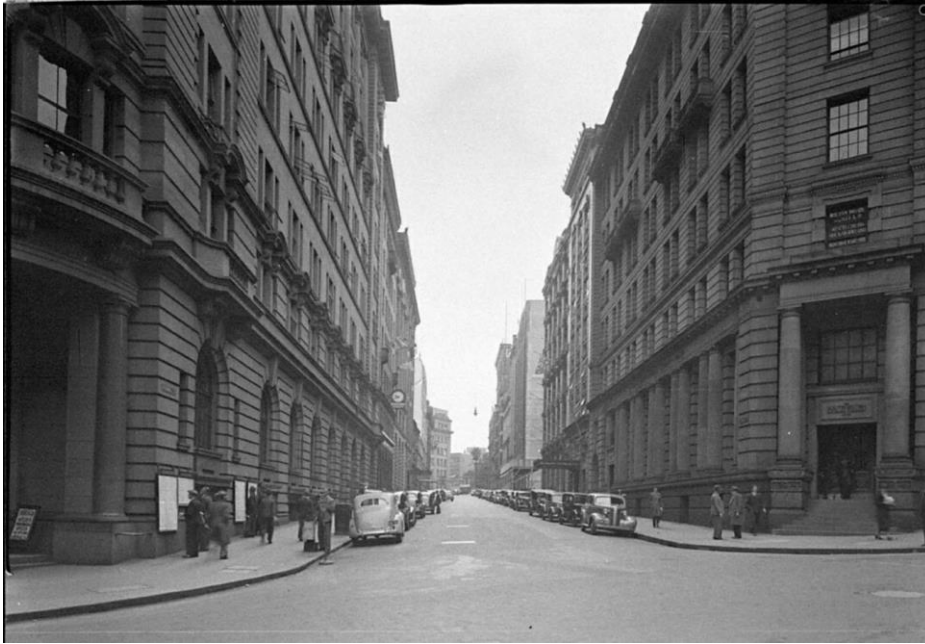
10 O'Connell Street in August 1938, view from Bent Street intersection. Source: SLNSW: Sam Hood, Home and Away – 9384, image FL1318558
