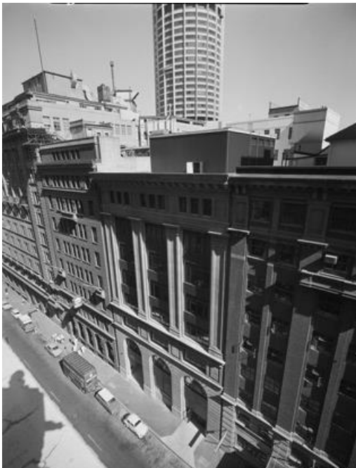
September 1971. The stair and lift housing on rooftop has been altered. Source: SLNSW: Max Dupain, Call no. ON 558/Box 82/nos. 580-594, contact sheet image 36537_10
