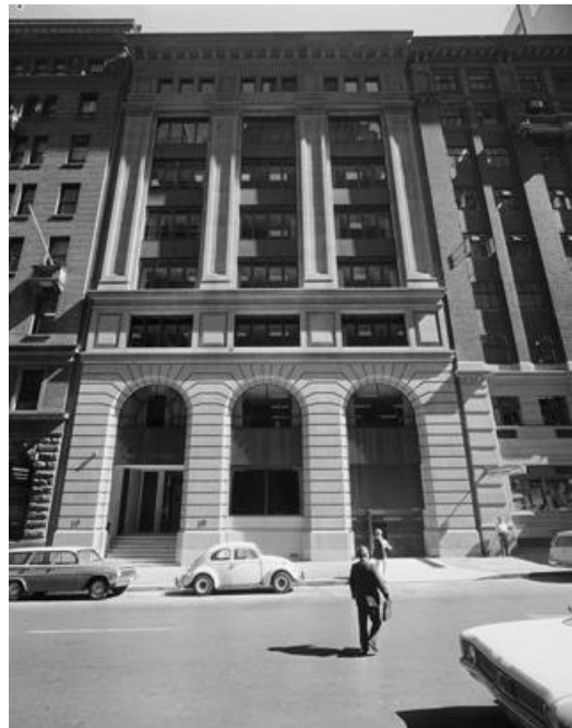
September 1971. The arch at right has been altered to provide driveway access to the new basement carparking. Source: SLNSW: Max Dupain, Call no. ON 558/Box 82/nos. 580-594, contact sheet image 36537_09
