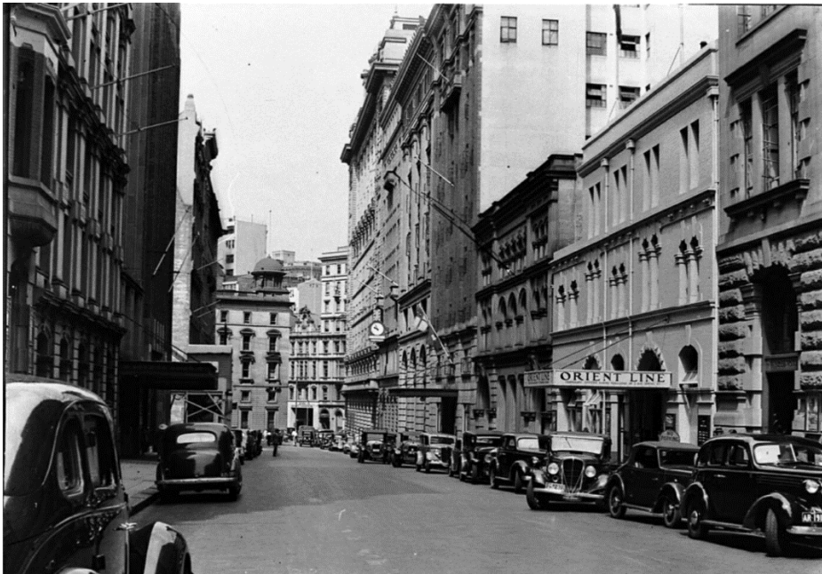
11 10-25 O'Connell Street; McKinsey House, Orient Steamship, 1939 Source: SLNSW: Hall & Co, Home and Away – 35225, image FL1643461
